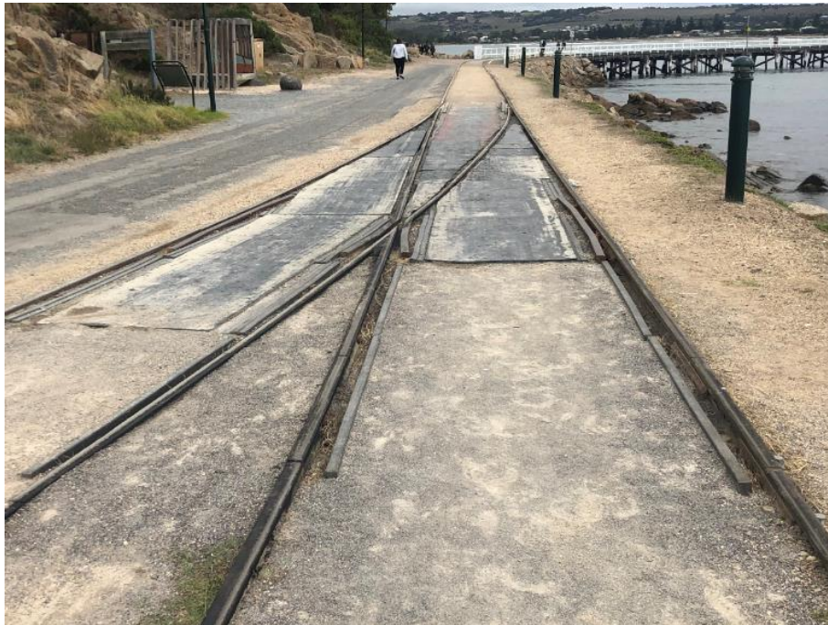
Figure 3.6: Typical Fixed Blade Turnout
