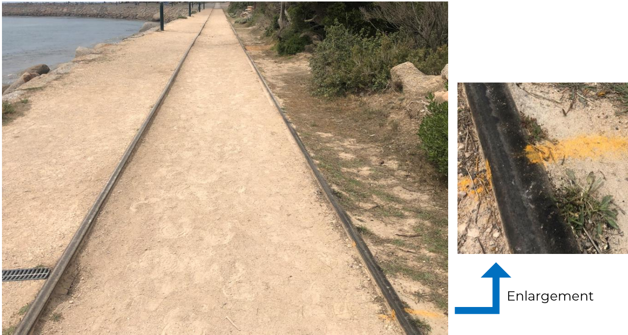
Figure 3.4: Typical Track on Granite Island with Marked Gauge Measurement Location
